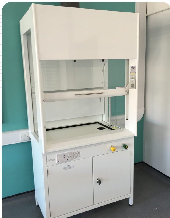
Fixed ducted fume cupboards for schools provide 100% exhaust to the atmosphere
